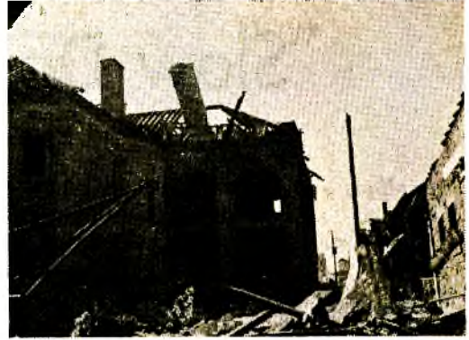
THE OLD GENERAL BOARD BUILDING gives way to the wrecker's sledge. The property was sold to the Novi Corporation of Detroit, who are erecting a new $125,000 regional office on the site.
