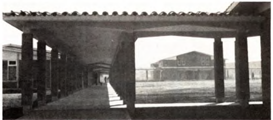
View of one side of the quadrangle on the new campus. The library is located to the left. To the right can be seen the auditorium.
